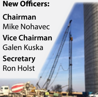
Construction is beginning on the new grain tube in Jansen. A huge post hole digger on this tall crane digs deep into the ground to form the pylons for the tank.
